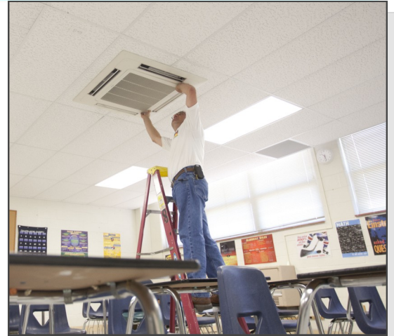
Bayless High School facility director Jeff Timeus inspects one of several Daikin VRV8, four-way ceiling mounted cassettes installed throughout the school.
