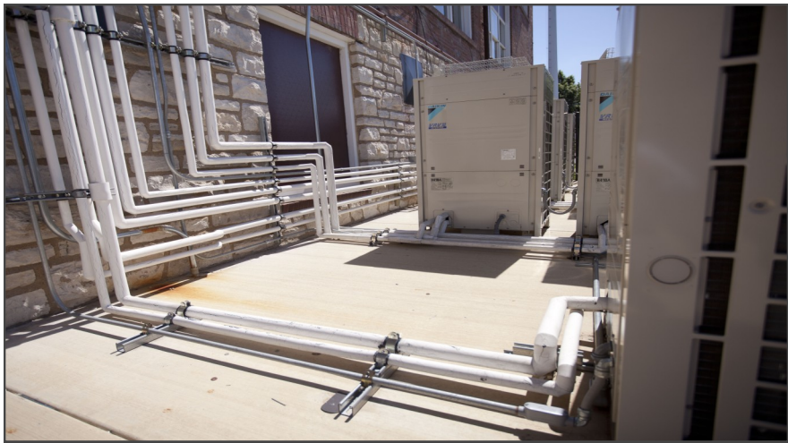
One key benefit is the Daikin VRV condensing units are relatively lightweight compared to traditional roof top units, they could be placed on the roof without compromising the roof structure.
